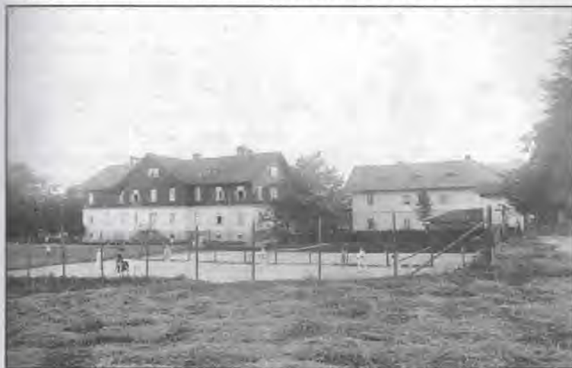
Schindlerovy domy, s.d.
